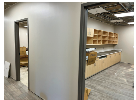
Work continues on the interior of the Special Learning Center’s school.
