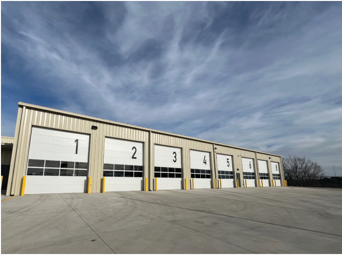
The new garage bay doors at CoMo Electric Sunrise Beach Operations Facility.
