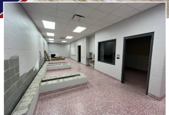
The new locker rooms are nearing completion.
