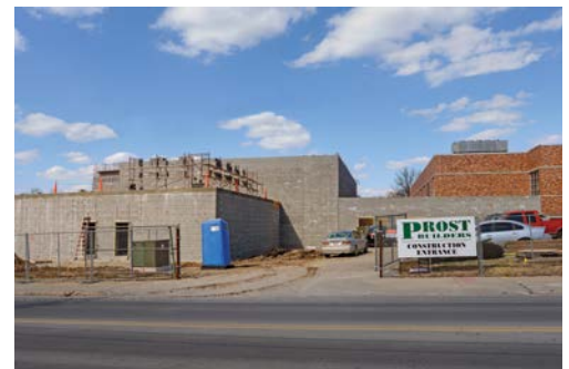
Jefferson Middle School locker rooms under construction.
