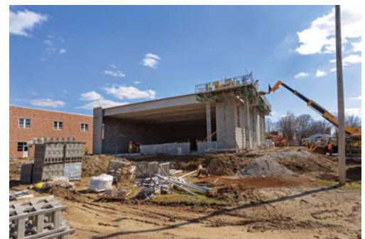
Jefferson Middle School gymnasium under construction.
